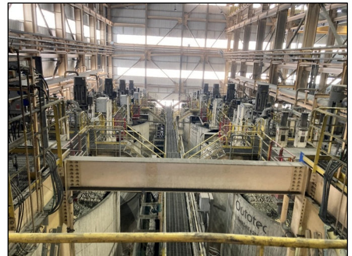
Figure 5. Rougher-scavenger in Copperton's concentrator, rows 7 and 8.
